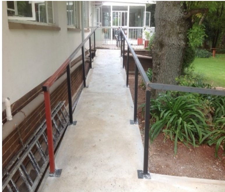
The Caro House wheelchair ramp progresses - start of installation of railings.
